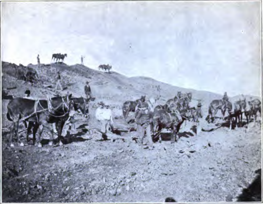
STRIPPING COAL AT LEHIGH, IND. T.
