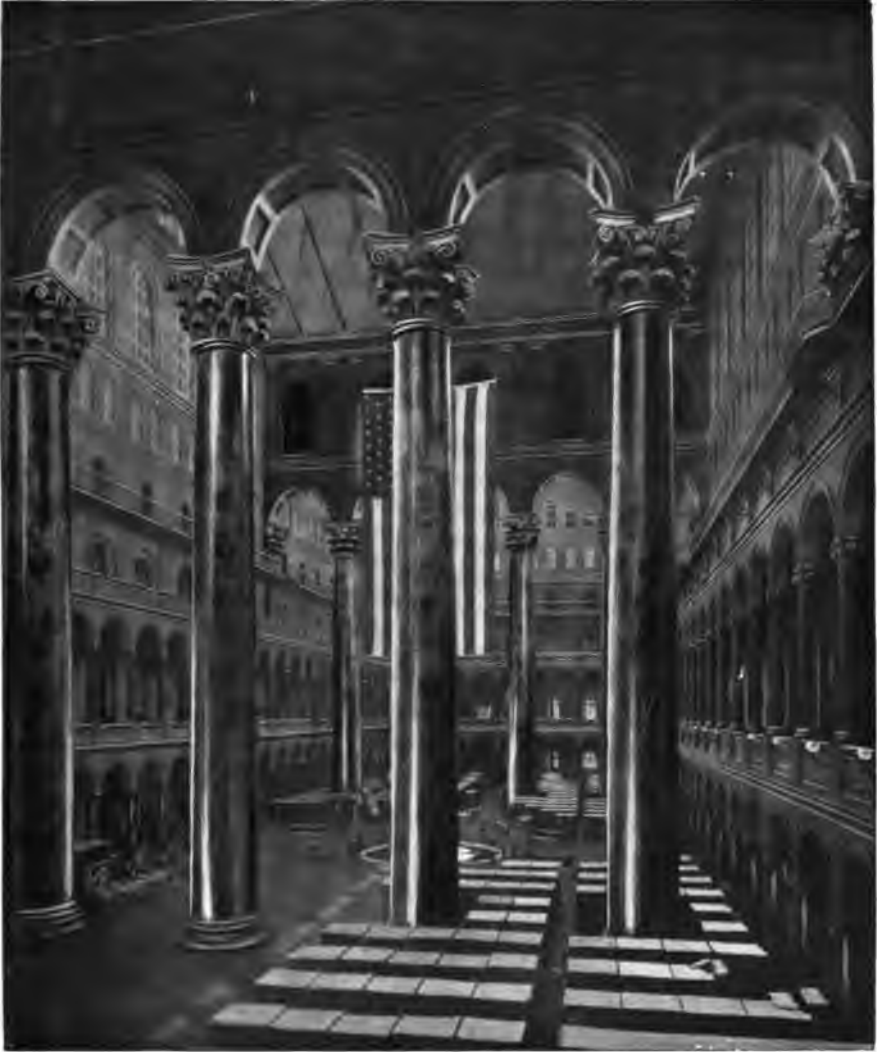
NORTH COURT OF GREAT HALL, PENSION BUILDING.
