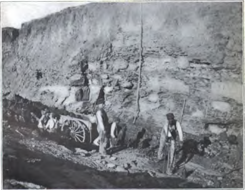
STRIPPING COAL AT LEHIGH, IND. T.
