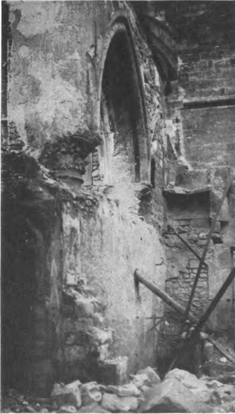
REDISCOVERED PORTION OF OLD CATHEDRAL CLOISTER, ABOUT WHICH A PARK IS TO BE ERECTED
