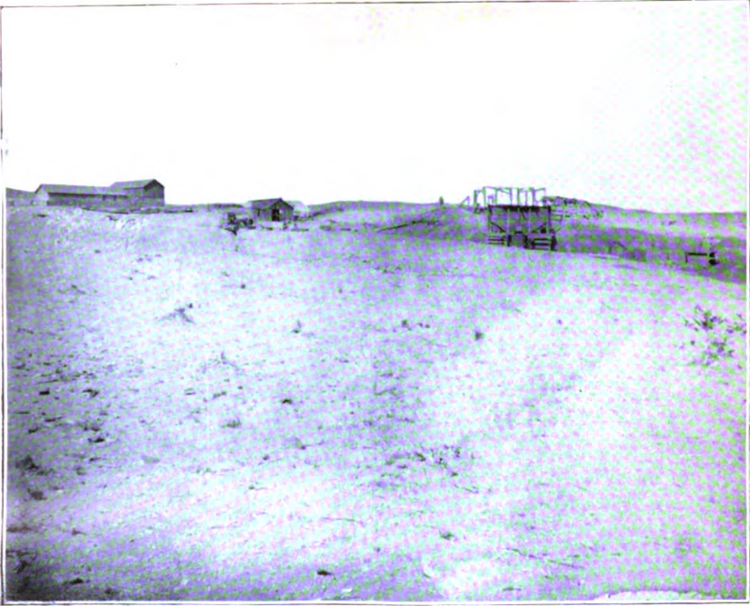
GENERAL VIEW CARTHAGE MINE NO. 3, 1900 AND 1901. Established and opened 1894.
