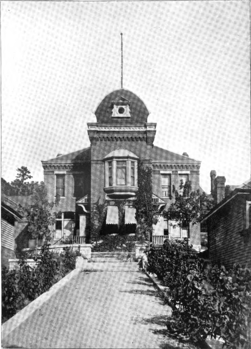
GOVERNMENT BATH HOUSE—FRONT VIEW FROM CENTRAL AVENUE.
