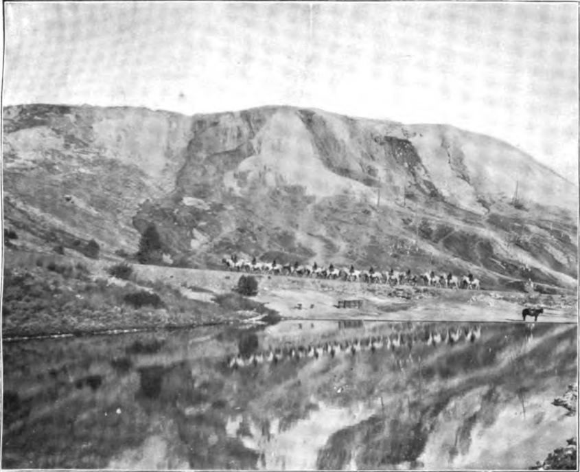
VIEW ALONG NEW RESERVOIR.
