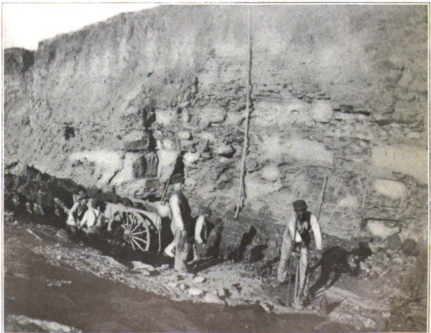
STRIPPING COAL AT LEHIGH, IND. T.
