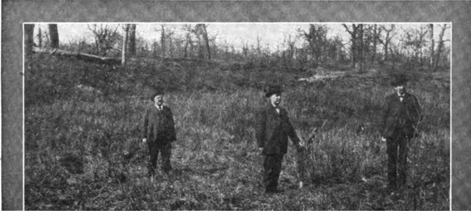
ABOUT TO BREAK GROUND AT GARY
