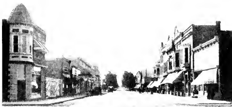
MAIN STREET, LOOKING SOUTH, KNOX
