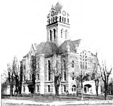
STARKE COUNTY COURTHOUSE, KNOX
