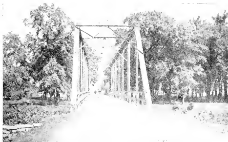
BRIDGE OVER YELLOW RIVER, KNOX
