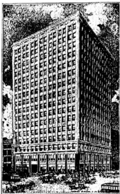
KIMBALL HALL BUILDING 308 So. Wabash Av. and Jackson Blvd.
