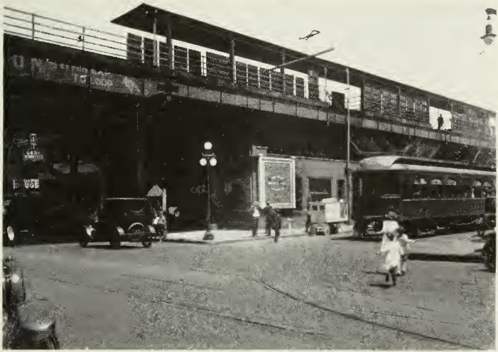
63rd and Halsted Where the Elevated R. R. and Interurban Meet
