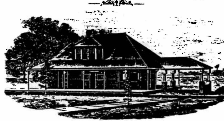
The original 95th Street Station, built c.1890, was replaced by the current structure in 1945.
