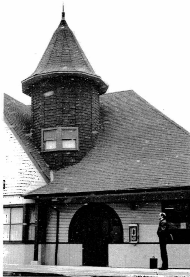
A 1889 drawing (left) of the 91st Street Station indicates the original Queen Anne-style details. Above, a contemporary photo of the station.
