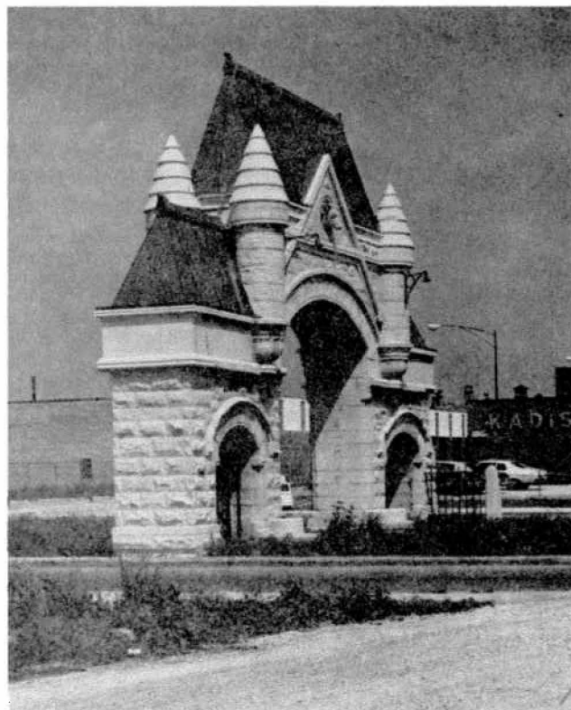
Southern wing (left) refinished with rusticated blocks and trim bands cut from the demolished guardhouse. (Barbara Crane, photographer)
