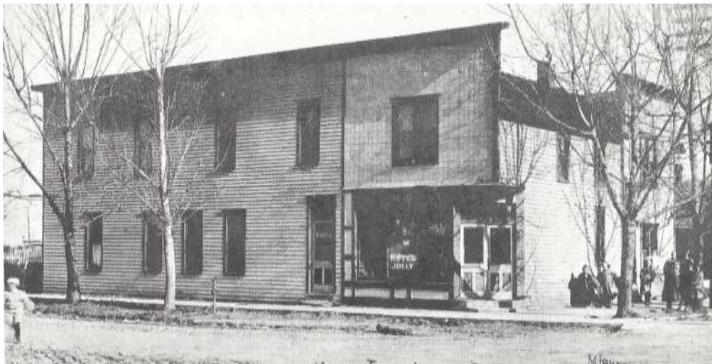
Northeast Corner Main and Davis Streets. Jolly Hotel, original part built in 1895.
