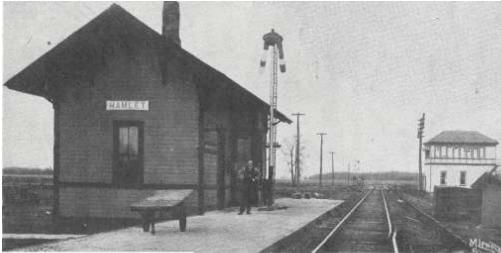
Original 3-1 depot built when railroad was completed (around 1895). Destroyed by fire in 1911. C. R. Lee, Agent.
