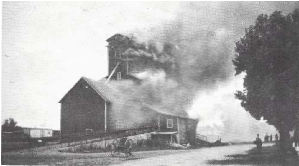
First elevator on Pennsy tracks. Built in 1900 by Hamlin Hardesty. Burned in June, 1915 when owned by Farmer's United Grain Co.
