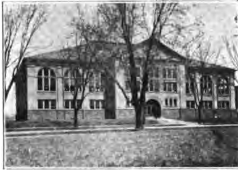
University of Illinois—Men's Gymnasium
