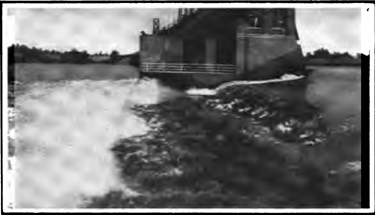
The Drainage Canal—The Bear Trap Dam, from Downstream
