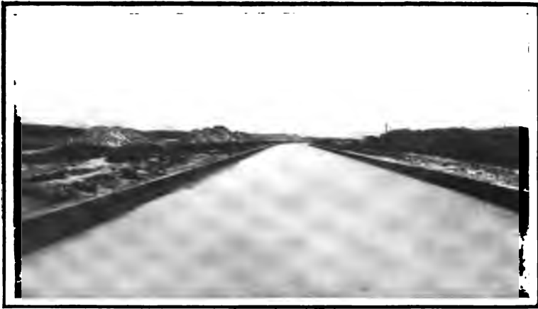
The Drainage Canal—Walls of Solid Stone Artificially Laid
