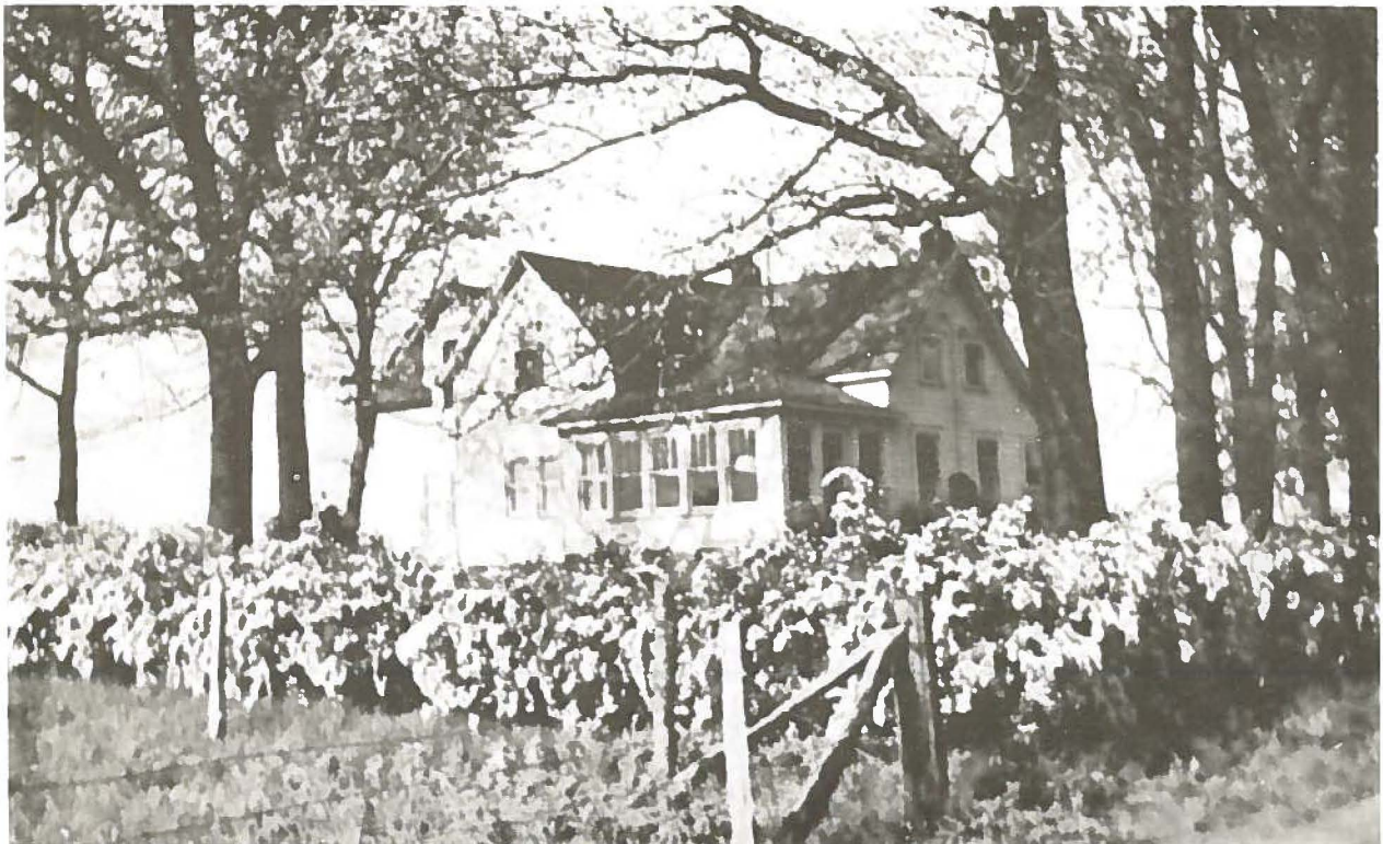
The same house after porch was removed and sun room added.
