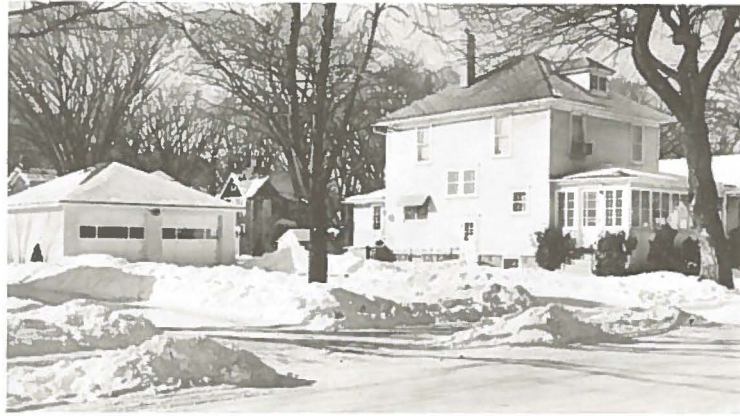
Larson Home—1917 to 1960 House removed intact to 1311 W. 10th St., Rock Falls
