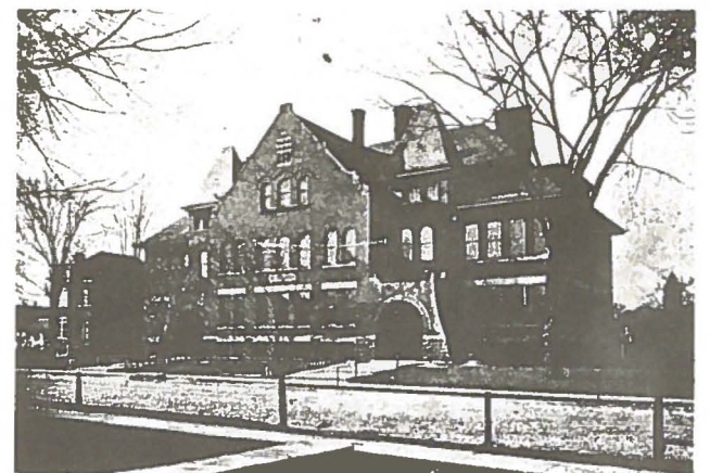
Sterling High School 5th Ave. between 4th and 5th Sts. Now removed
